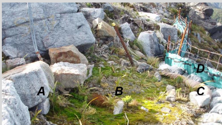
Figure C33. A range of soil-retaining and buffer-creating practices to protect adjacent ecosystems along a steep ridgeline, Stockton Mine. A: Barrier of large boulders; B: planted seedlings; C: Erosion 'log'; D: Sediment/silt fence. Slow-release fertiliser was used to stimulate cover of mosses (which were already present, but sparse).
