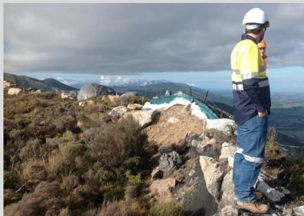
Figure C33. A range of soil-retaining and buffer-creating practices to protect adjacent ecosystems along a steep ridgeline, Stockton Mine. A: Barrier of large boulders; B: planted seedlings; C: Erosion 'log'; D: Sediment/silt fence. Slow-release fertiliser was used to stimulate cover of mosses (which were already present, but sparse).
