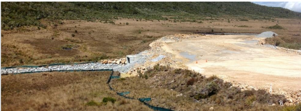
Figure C35. Construction of the Cypress mine haul road. The steep road batters are covered with sods of tussock, mānuka and wire-rush. These immediately provide sediment control and buffering.
