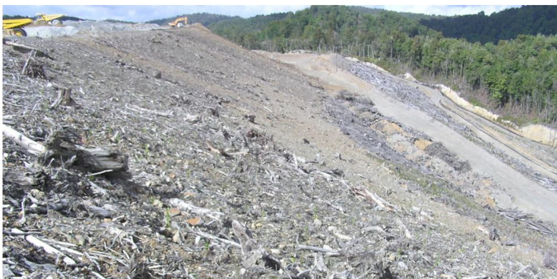
Figure 26. Slash spread across backfilled slopes reduces the risk of erosion.
