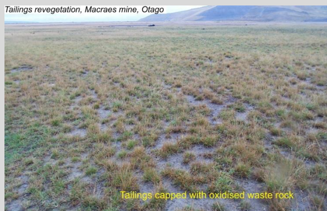
Figure C40. Revegetation of decommissioned tailings capped with oxidised waste rock initiated using pasture grasses and fertiliser.
