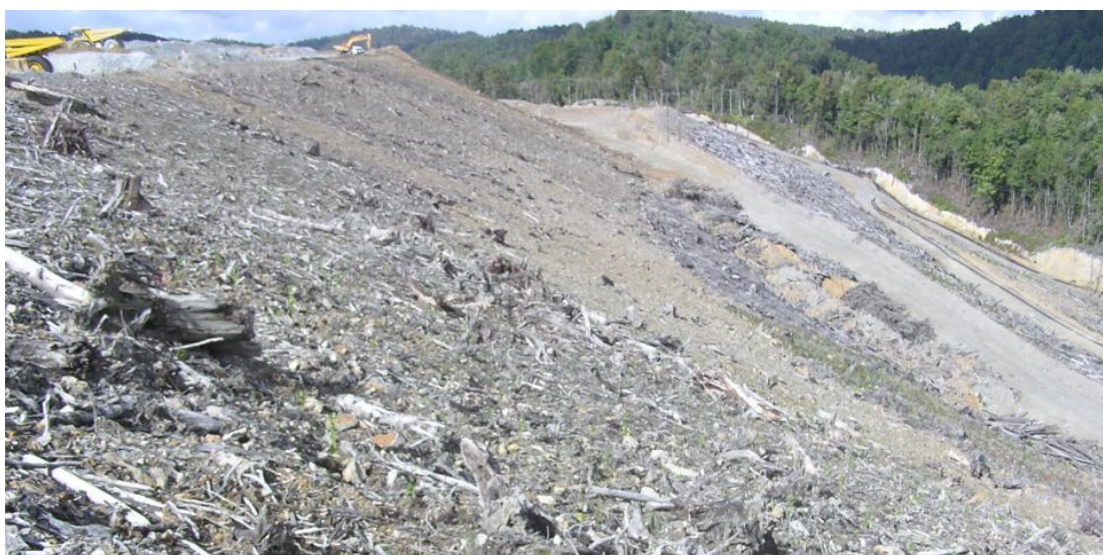
Figure 32. Slash spread across backfilled slopes reduces the risk of erosion.
