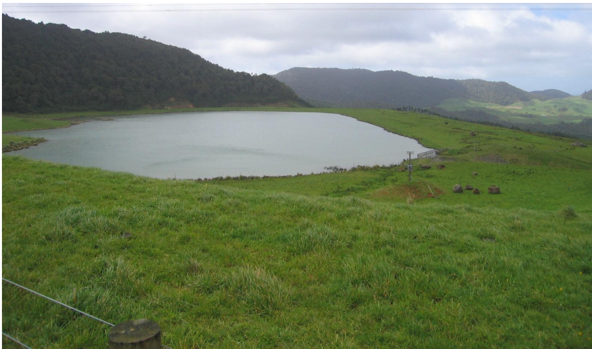
Figure 17. Water cover over tailings storage facility at Golden Cross mine site. NAF rock was used for surface rehabilitation, and pasture was planted for a farming operation.
