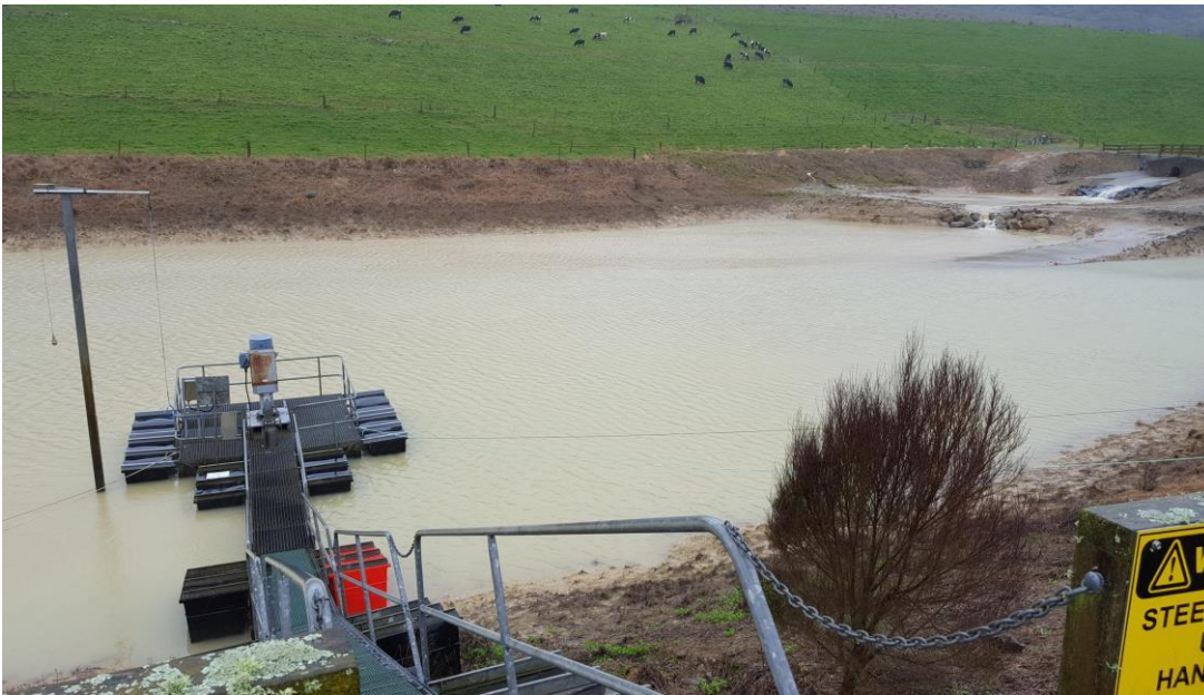
Figure 31. Sediment control pond at Waihi mine. Water quality is continuously monitored, and when water chemistry (pH, EC and turbidity) is appropriate, this pond can be discharged directly. At other times it reports to the water treatment plant.
