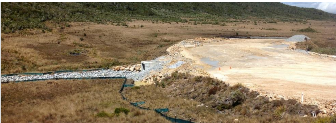
Figure C33. Construction of the Cypress Mine haul road. The steep road batters are covered with sods of tussock, mānuka and wire-rush. These immediately provide sediment control and buffering.
