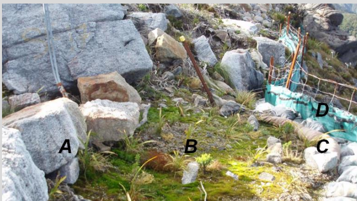
Figure C32. A range of soil-retaining and buffer-creating practices to protect adjacent ecosystems along a steep ridgeline, Stockton Mine. A: Barrier of large boulders; B: planted seedlings; C: Erosion 'log'; D: Sediment/silt fence. Slow-release fertiliser was used to stimulate cover of mosses (which were already present, but sparse).
