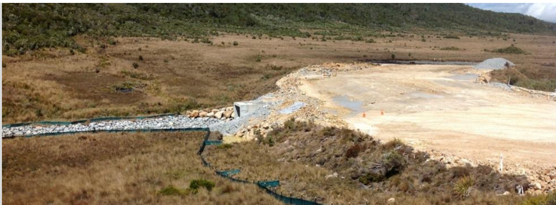
Figure C29. Construction of the Cypress Mine haul road. The steep road batters are covered with sods of tussock, mānuka and wire-rush. These immediately provide sediment control and buffering.
