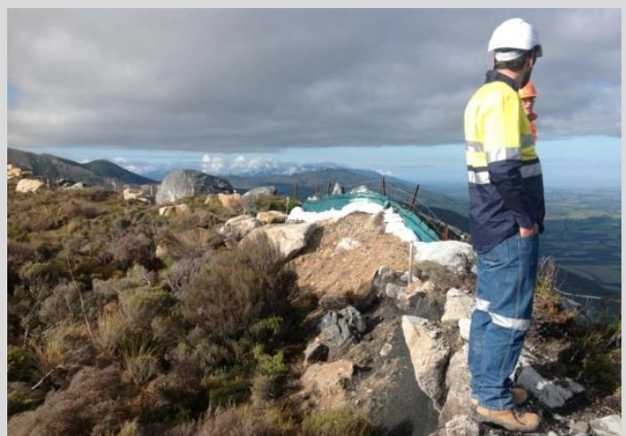
Figure C27. A range of soil-retaining and buffer-creating practices to protect adjacent ecosystems along a steep ridgeline, Stockton Mine. A: Barrier of large boulders; B: planted seedlings; C: Erosion 'log'; D: Sediment/silt fence. Slow-release fertiliser was used to stimulate cover of mosses (which were already present, but sparse).
