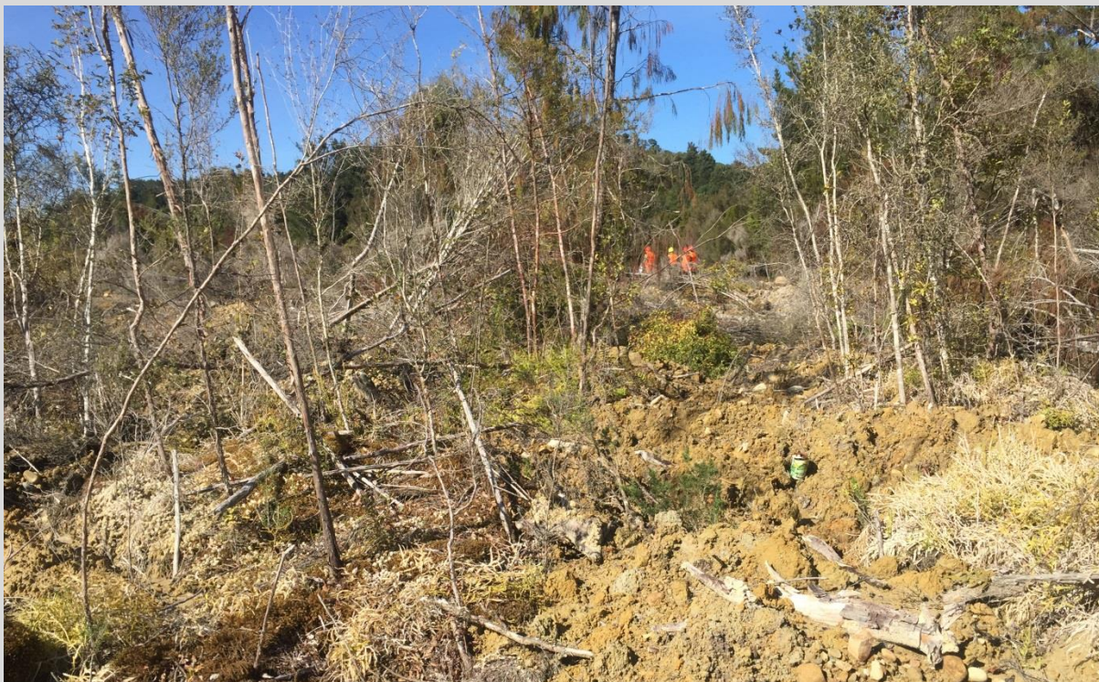
Figure C24 Effective, young direct transfer. Note the high proportion of intact leaf litter, many upright saplings, and soil placed around and between sods to help protect them from drying out and keep them upright.
