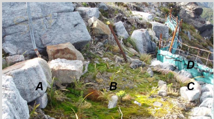
Figure C27. A range of soil-retaining and buffer-creating practices to protect adjacent ecosystems along a steep ridgeline, Stockton Mine. A: Barrier of large boulders; B: planted seedlings; C: Erosion 'log'; D: Sediment/silt fence. Slow-release fertiliser was used to stimulate cover of mosses (which were already present, but sparse).
