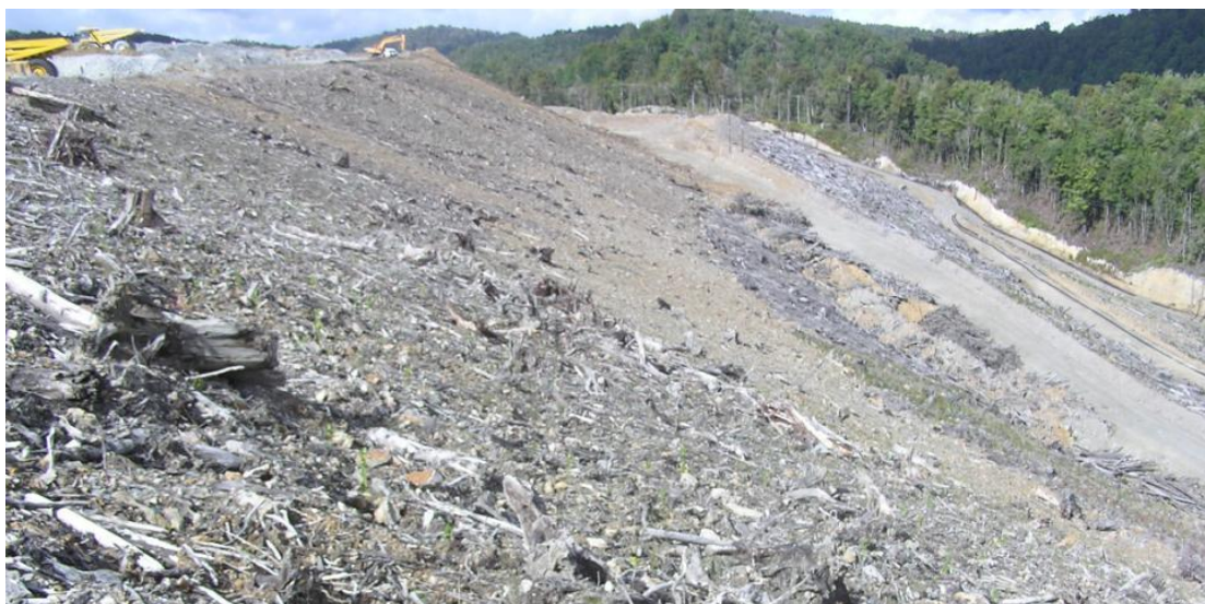
Figure 33: Slash spread across backfilled slopes reduces the risk of erosion.
