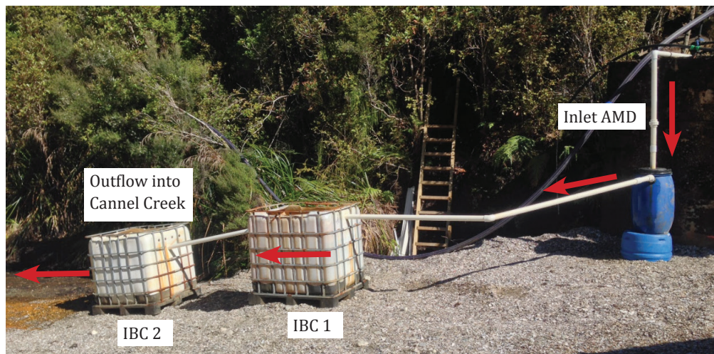
Figure 3 Diversion well setup at Bellvue Mine site. Inlet AMD enters the well where fluidization of substrate occurs. Treated water then flows through each IBC, where further dissolution of substrate and neutralisation reactions occur. Treated water then flows into Cannel Creek.
